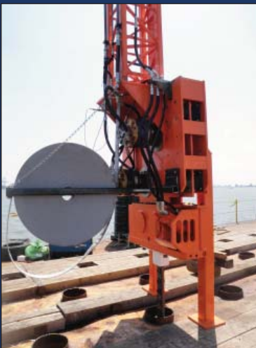
One roll of wick drains can be as much as 1,000 feet long.
