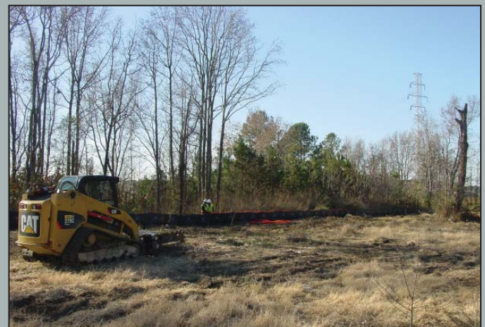
Workers prepare for construction by placing tree protection fencing around the Paradise Creek site to prevent erosion.
