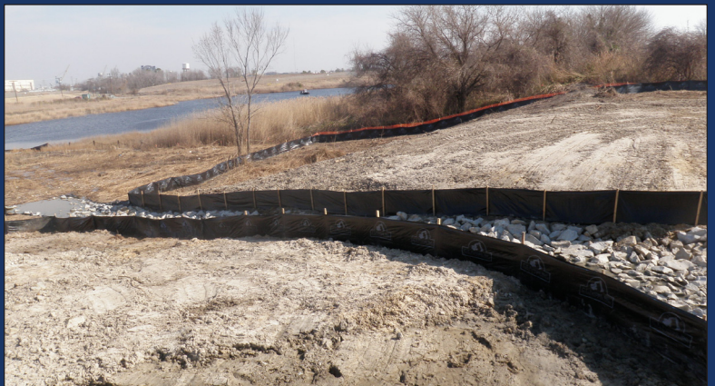
Erosion control measures, such as the water detention basin (above) and rip-rap lined channel (below), will ensure that trees surrounding Paradise Creek will not be damaged as the land is excavated and replaced with healthy wetlands.
