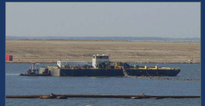
A floating pipe moves the sand from the Liberty Island dredge to the spill barge as it places sand along the division dike's footprint.
