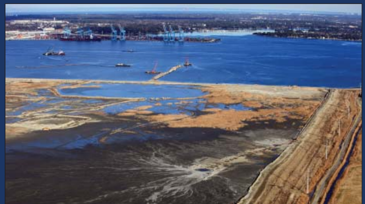
This aerial view of the CIDMMA shows the containment cells that are used to allow the sediment to settle, so that only clear water is returned to the river.
