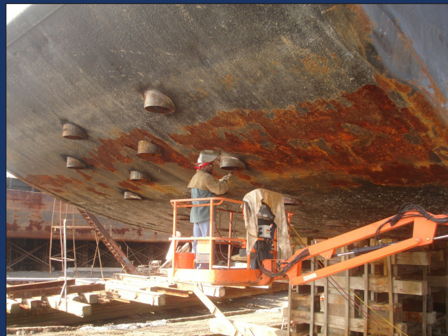
A worker welds pipes into the barge in the pattern that the PVDs will be installed. This template will help the contractors guide the PVDs into the correct position underwater without having to reposition the barge.
