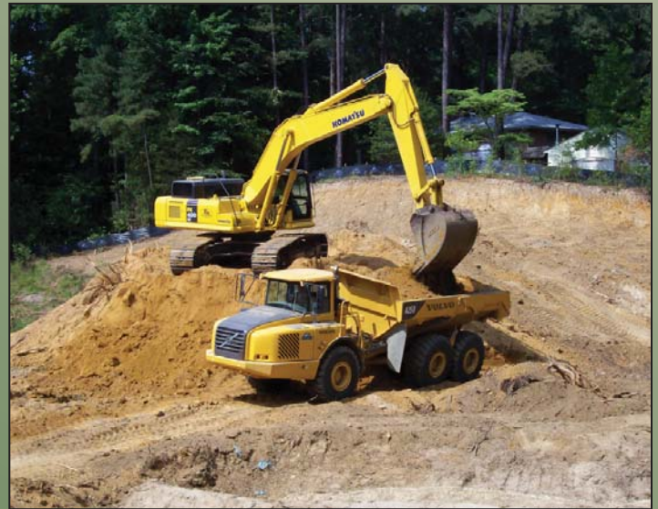
Excavators will be used for bulk dirt removal at the site.
