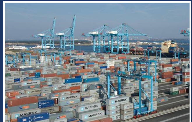
APM Terminals is fully-automated and the most technologically advanced marine terminal on the east coast. The terminal has six cranes, six on-dock rail tracks, and a capacity of 1 million TEUs.
