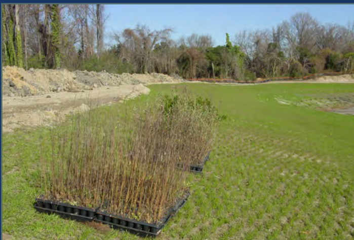
Currently, the upper "high marsh," or lower slope, of the site is being planted with shrubs which will remain dormant for the winter.
