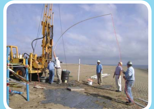
Piezometer Installation
