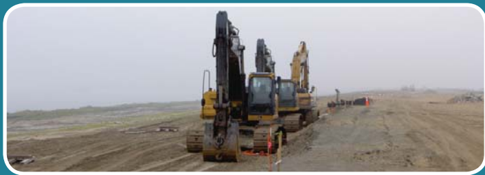
Trackhoes Are Shown Along The North End Of The Berm
